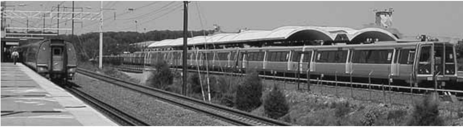
Both the high-level Amtrak (left) and Metro (right) New Carrollton stations can be seen
