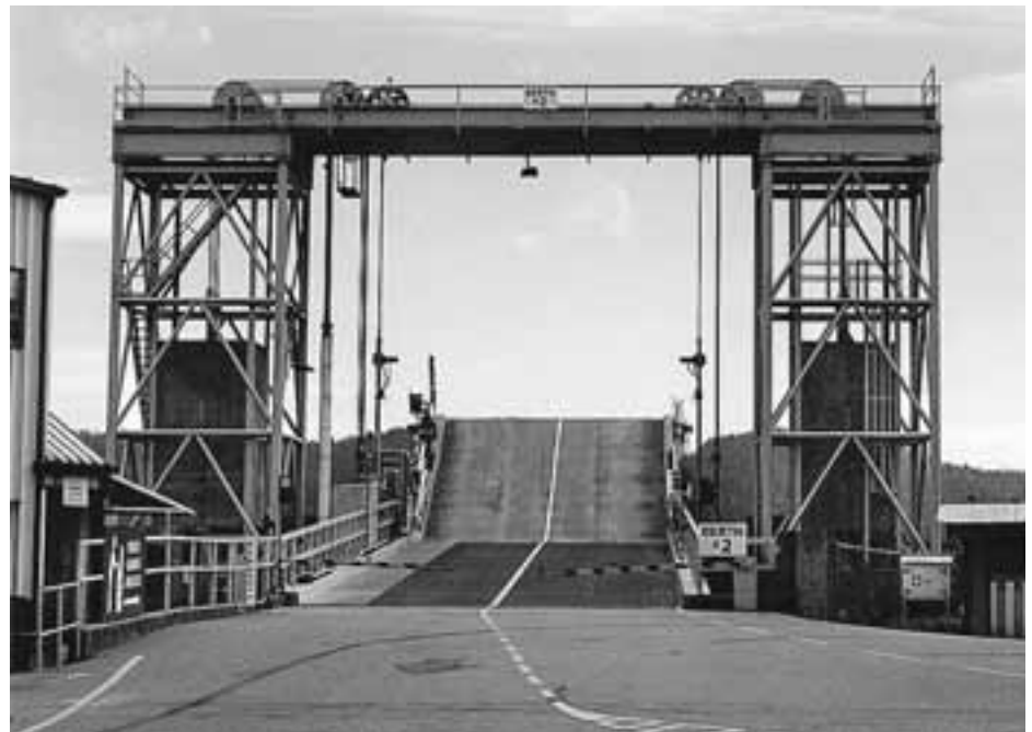
The relationship of the two outer tower and the horizontal bridge is depicted by this shot of the Langsdale slip on the Sunshine coast near Gibson's. This slip would appear to support one ramp only, and is the closest to the interpretation suggested by this article. Notice also that this slip features an internal stairway, while others have vertical ladders. (Tom Patterson photo)
