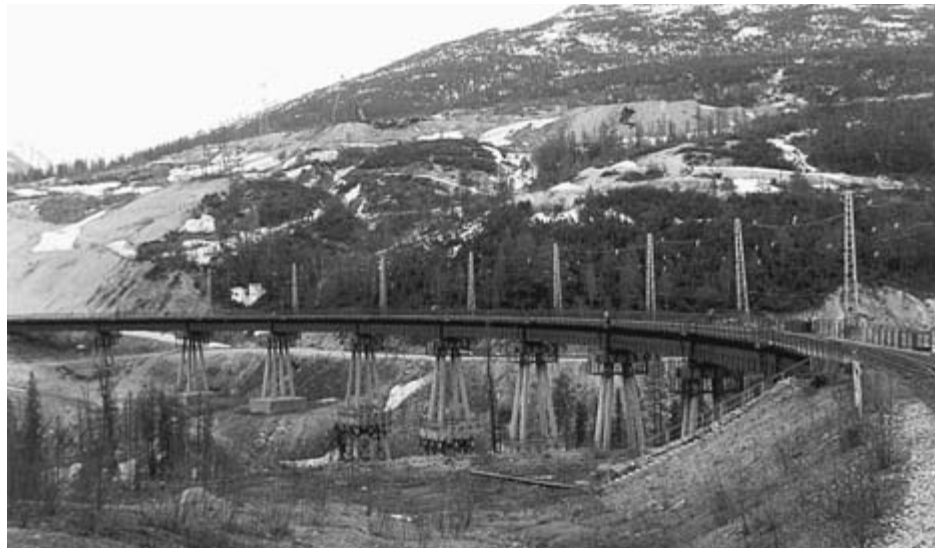
Chertov Bridge on the BAM.
