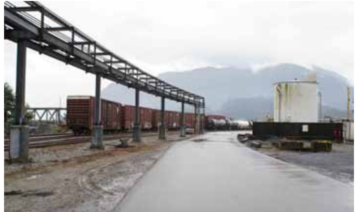
Photo 1: This view of the inbound and outbound tracks at the Howe Sound mill illustrates the predominate kind and volume of freight cars used, namely box and tank cars. For this mill, all inbound and outbound traffic travelled by water. Wood chips are ferried by barge.
