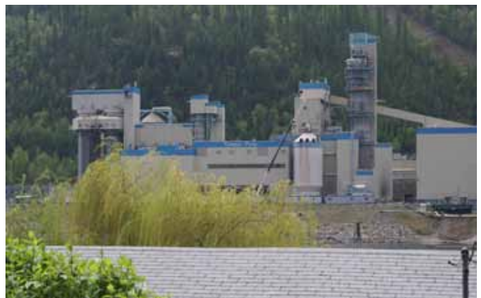
Photo 2: It is very difficult to encompass an entire mill in one photograph. This "far-away" view of the south end of the Celgar mill at Castlegar, BC, is an attempt to do so.
