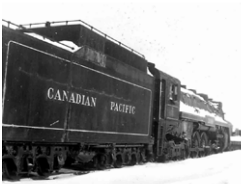
#3100 on "hold" at the Weston Shops
