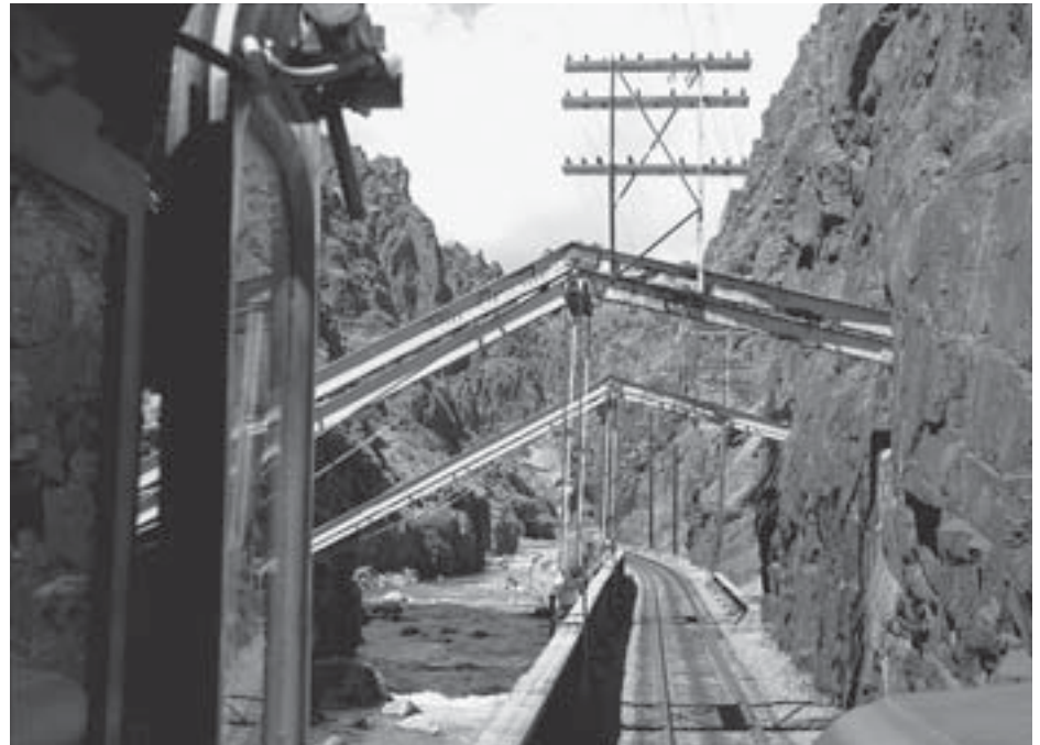
This particular bridge on the D&RGW inspired Normand Levert to build a hanging “S” curve tunnel to connect his NORD to his staging yard.
