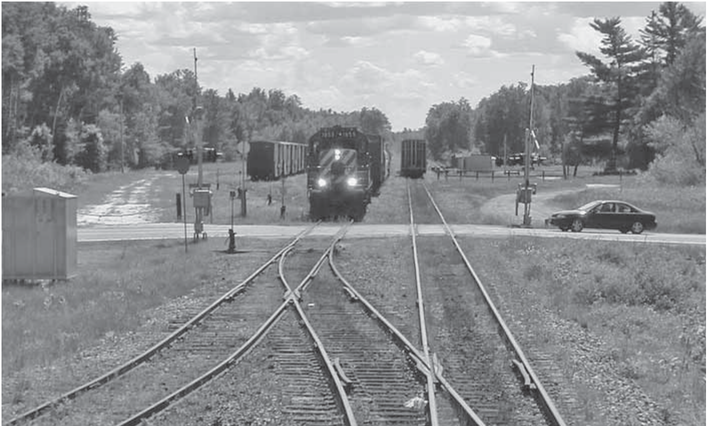
OCR train works the compact four-track yard at Portage du Fort.
